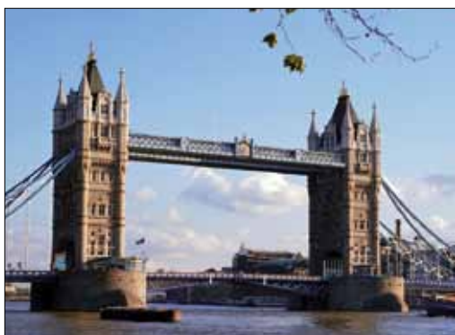
Tower híd, London Tower Bridge, London
